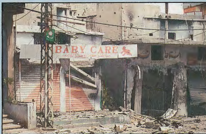
Most houses in the region are simply built of concrete slabs: RPGs, TOWs and small arms fire do no more damage than leave entry and exit holes. 155 HE rounds and 2,000-pound bombs, however, will change a village beyond recognition. Photo: Jim Marks
